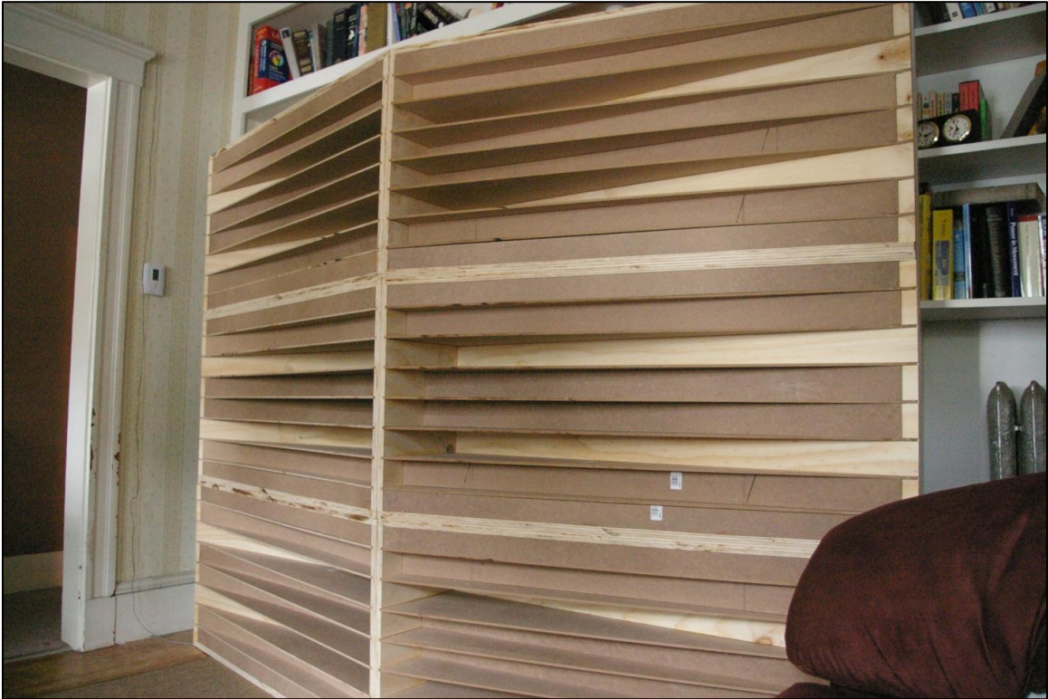
Figure 12 Horizontally oriented array of six p=7 acoustic ramp diffusers.
